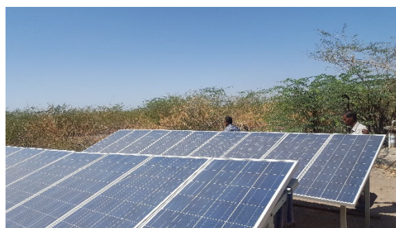
Solar panels installed at a water supply scheme in Afar region. Photo Credit: Lowland WASH Team.
