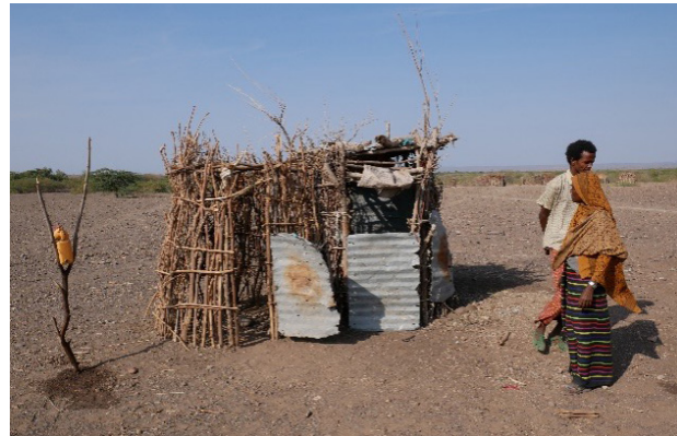
A tippy tap and household latrine constructed from locally available materials in sangumare kebele, araso woreda, somali region. Photo credit: Fostvedt-Mills Consulting.
