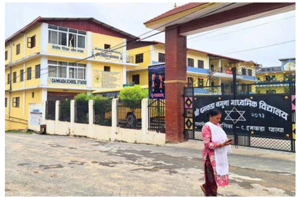
Pedestrian using the road upgraded by LISP in front of the Damkada Secondary School
