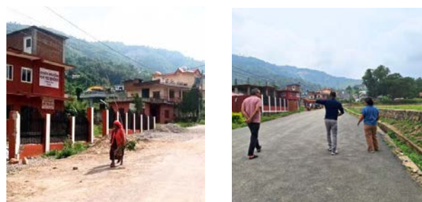
Picture of the road upgradation before (left) and after (right)
